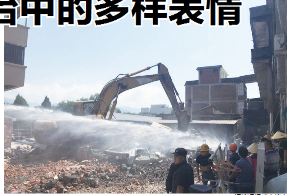
拆违现场喷水抑尘
